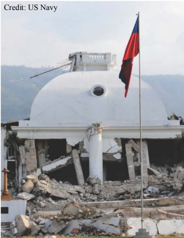
Figure 6-1: The Collapsed Presidential Palace of Haiti
